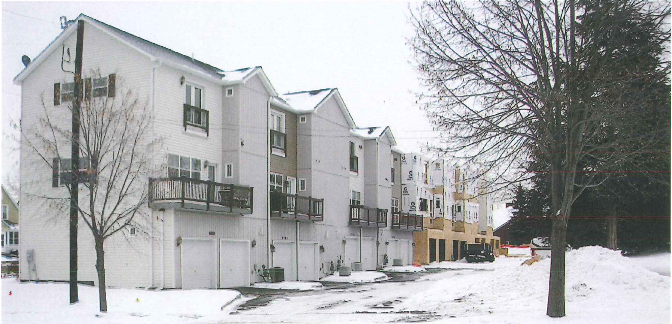
Across Bradford from parking lot
