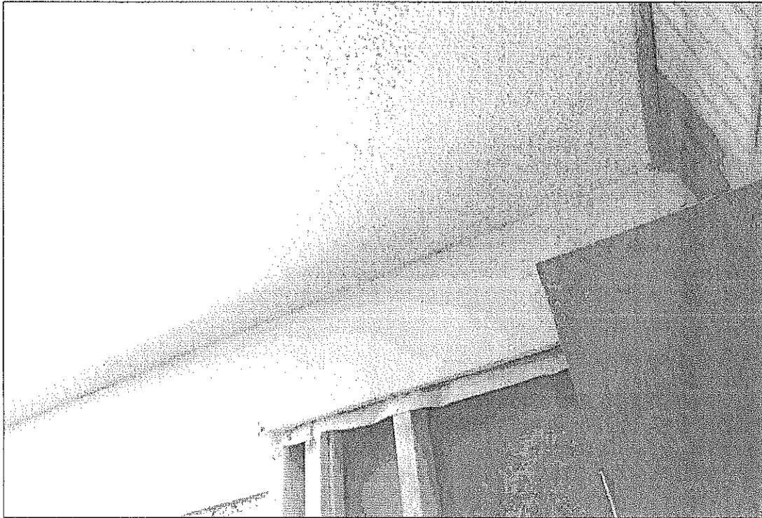
**Photograph # 16:** Water stains at wall/ceiling
