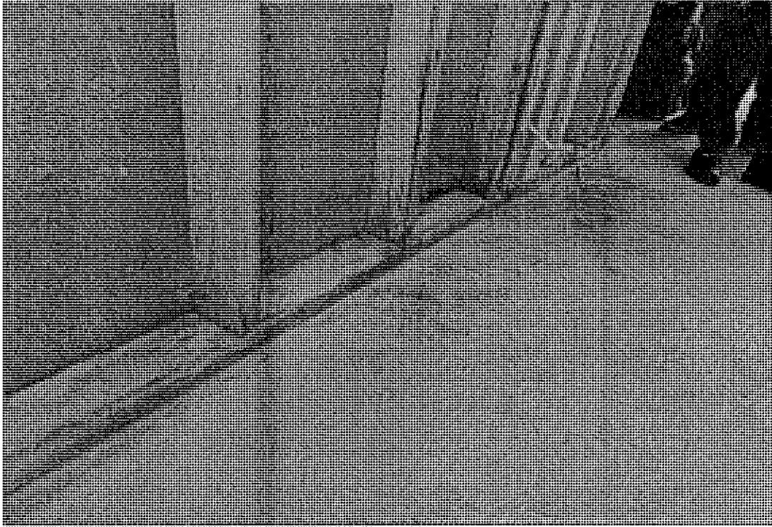
**Photograph # 3:** Staining on floor below the window in Photo 1
