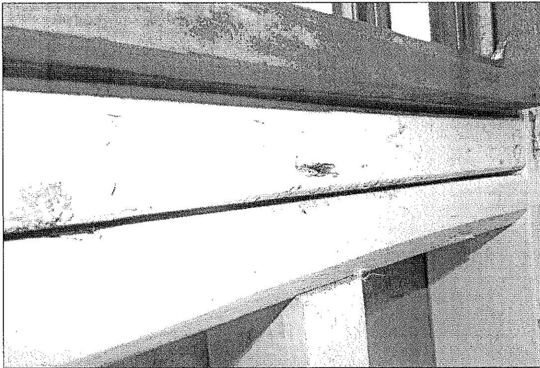
**Photograph # 24:** No flashing below window
