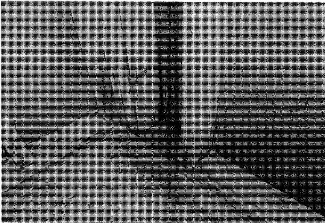
**Photograph # 5:** Close up of water staining below window in Photo 4
