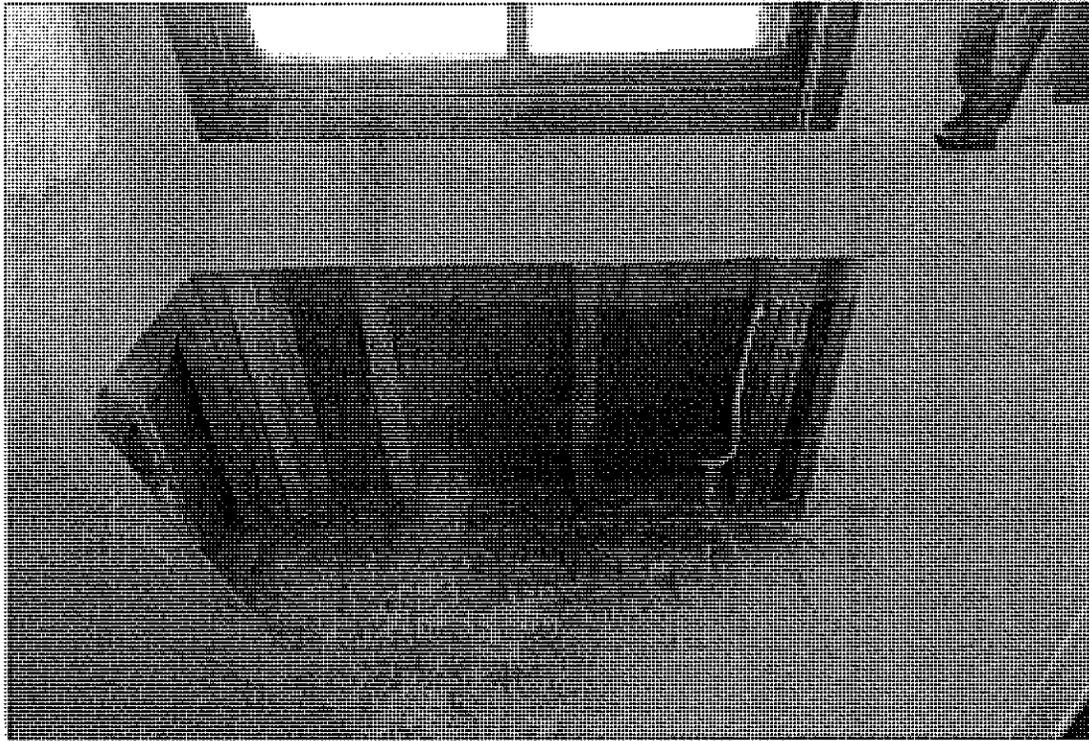
**Photograph # 4:** Water staining on floor below window to the west
