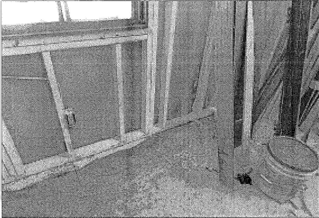
**Photograph # 11:** Bedroom – water staining on floor; Kilz applied to wall
