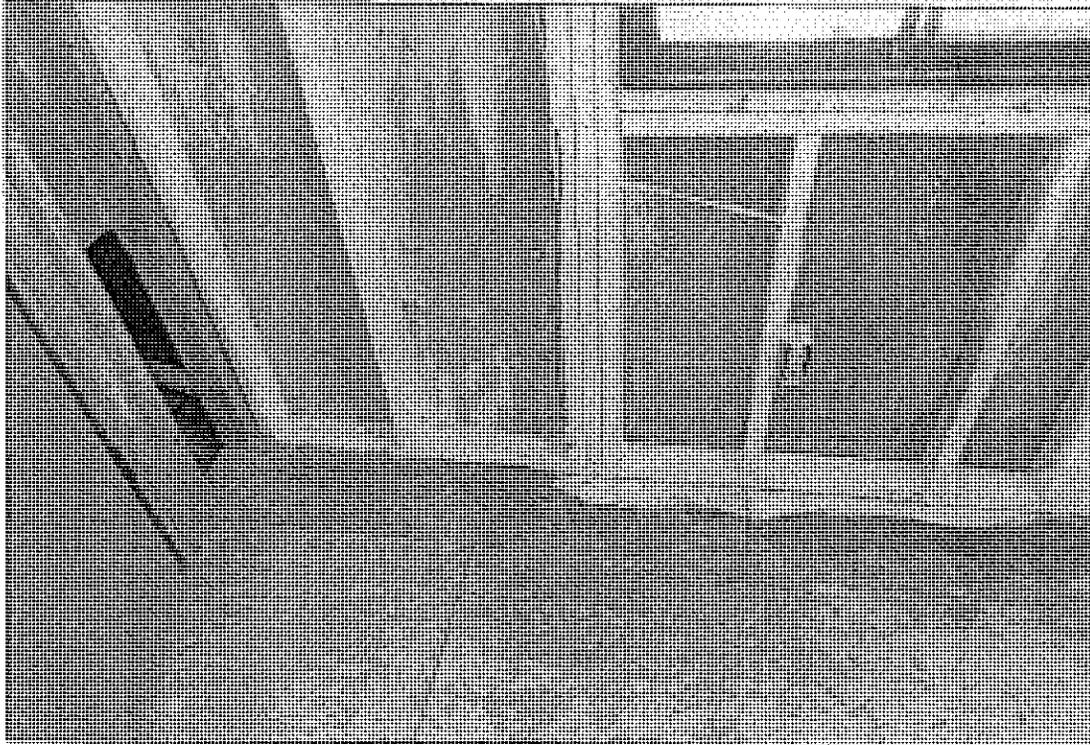
**Photograph # 10:** Bedroom – water staining on floor; Kilz applied to wall
