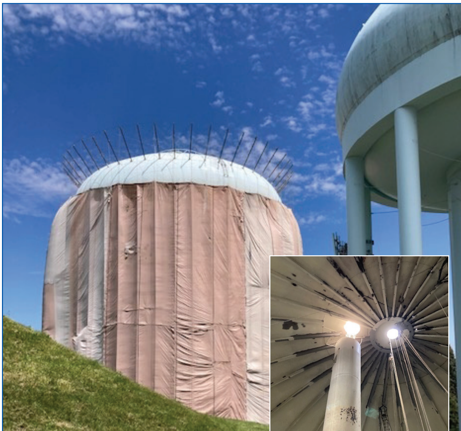
Highland water tank No. 2 gets sandblasted as part of the preparation for a new coat of paint gets underway on May 23. Photos by Todd Blomstrom.
