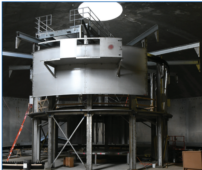
The inside of the clarifier on a tour of the new treatment plant held on May 24.
