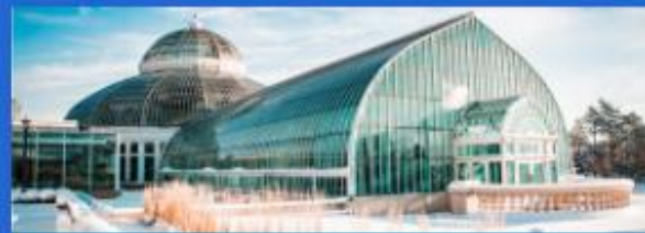
City Buildings and Operations
