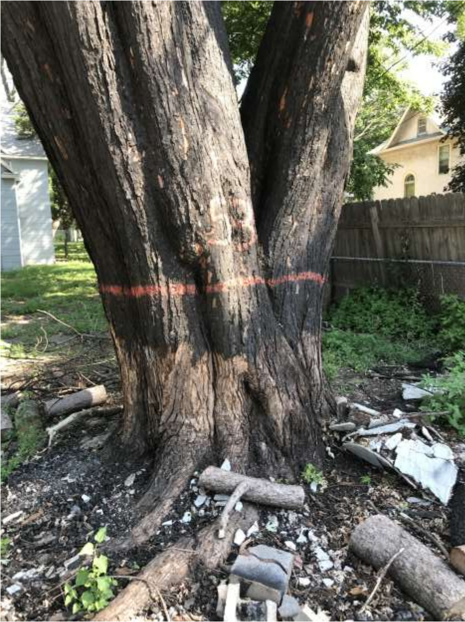
1672 Taylor Ave – Burned Tree Close Up 8-23-22
