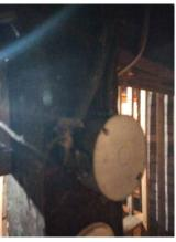
6. Box not sercure to wall, required to attach box securly to wall.
