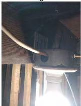
2. Box required for light fixture in basement.
