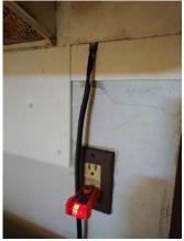
12. Outlets without grounding, require GFCI/AFCI device and "No Equipment Ground" Label on device.
