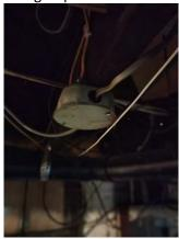
11. Hood power cord improperly installed, risk of shorting circuit. Requires dedicated hood circuit and accesable outlet or hard wiring of hood.
