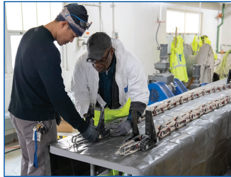
Panha Chan and Arnett Hughley work on repairing chains from clarifier 3.
