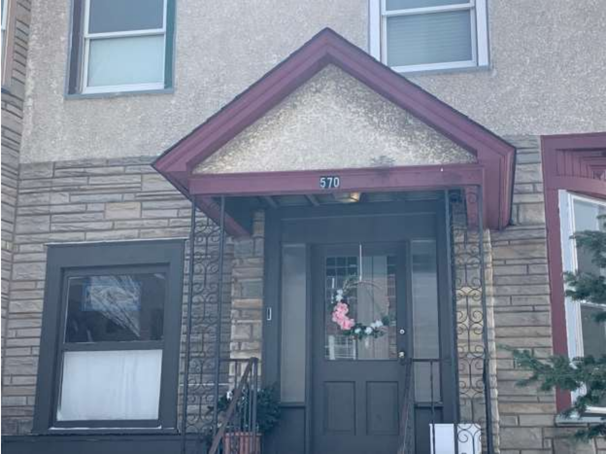
570 Portland Ave. Photo 3-17-23
