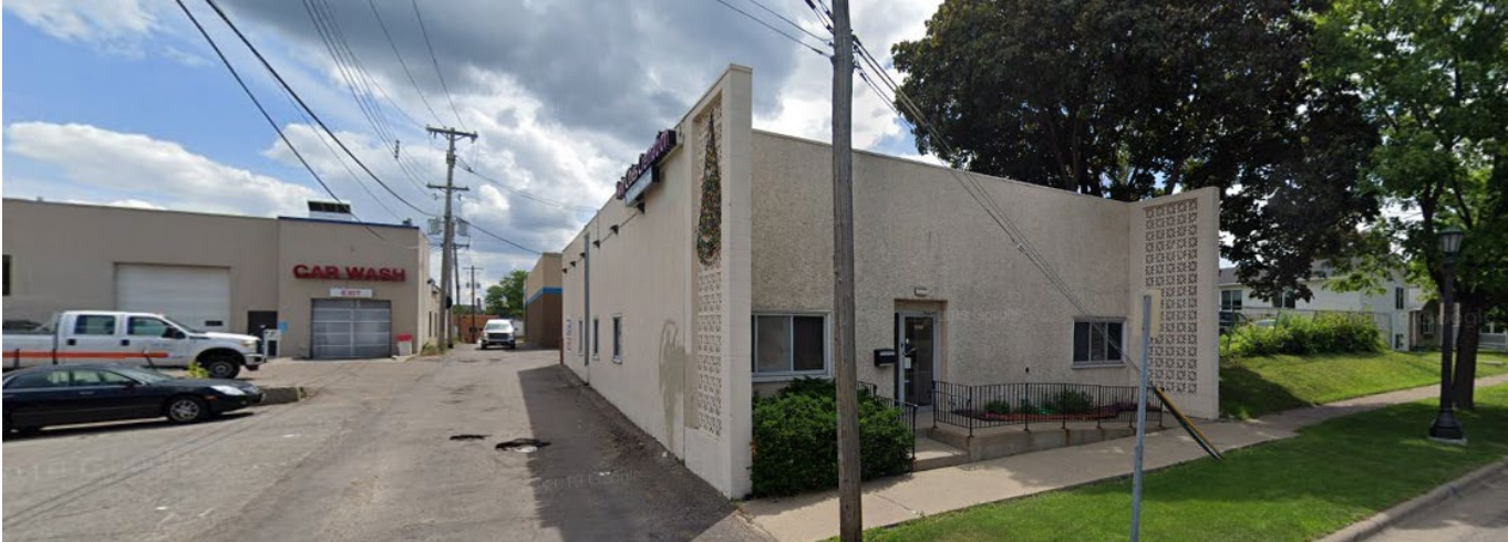
1598 Carroll Avenue in a T2 district and abutting alley to the east
