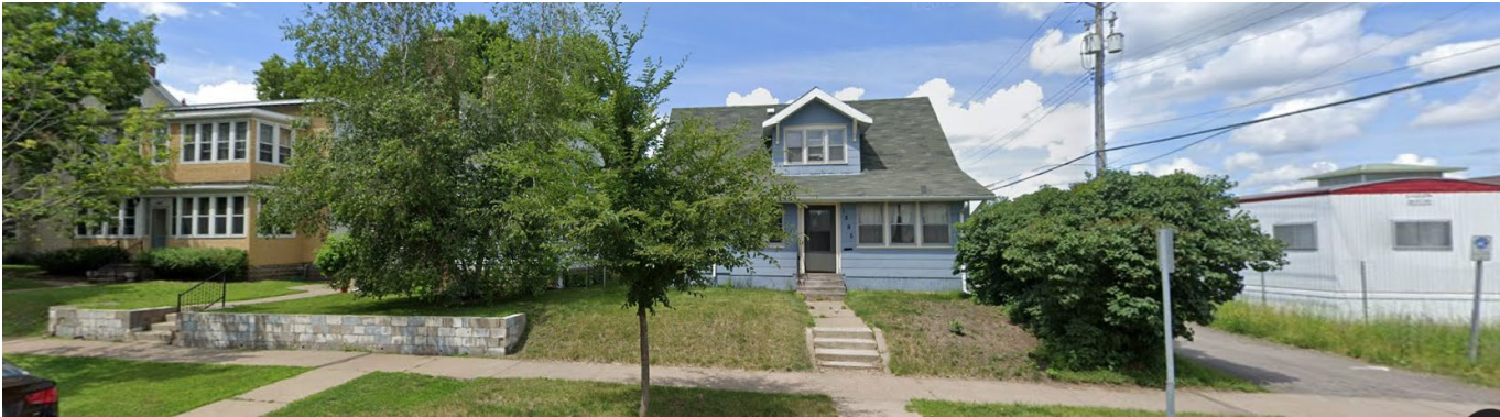
One and two-family homes north side of Carroll Avenue in RT1 district
