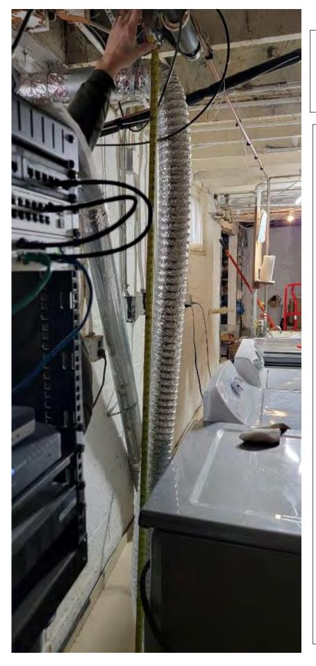
Dryer exhaust vent: Current transition duct length is ~79" It connects to solid metal ductwork at the dryer and to the outside connection.
