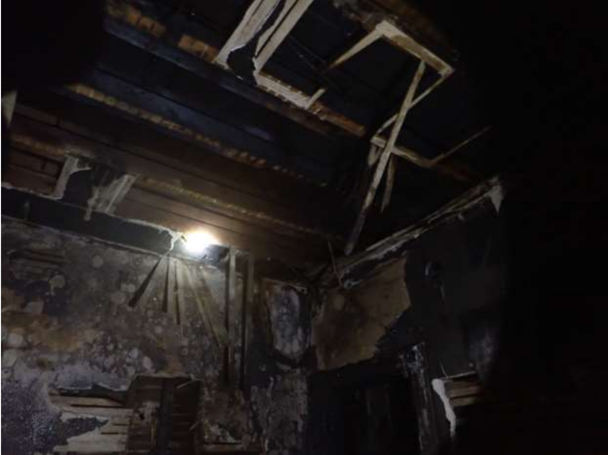
326 Charles Ave – Fire photos sent on 7/11/23
