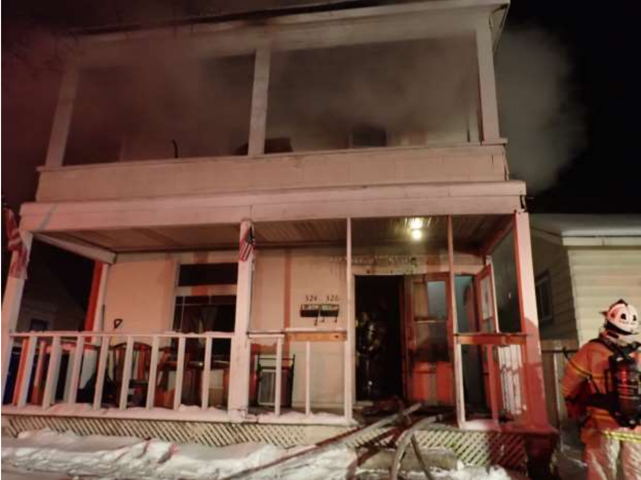
326 Charles Ave – Fire photos sent on 7/11/23
