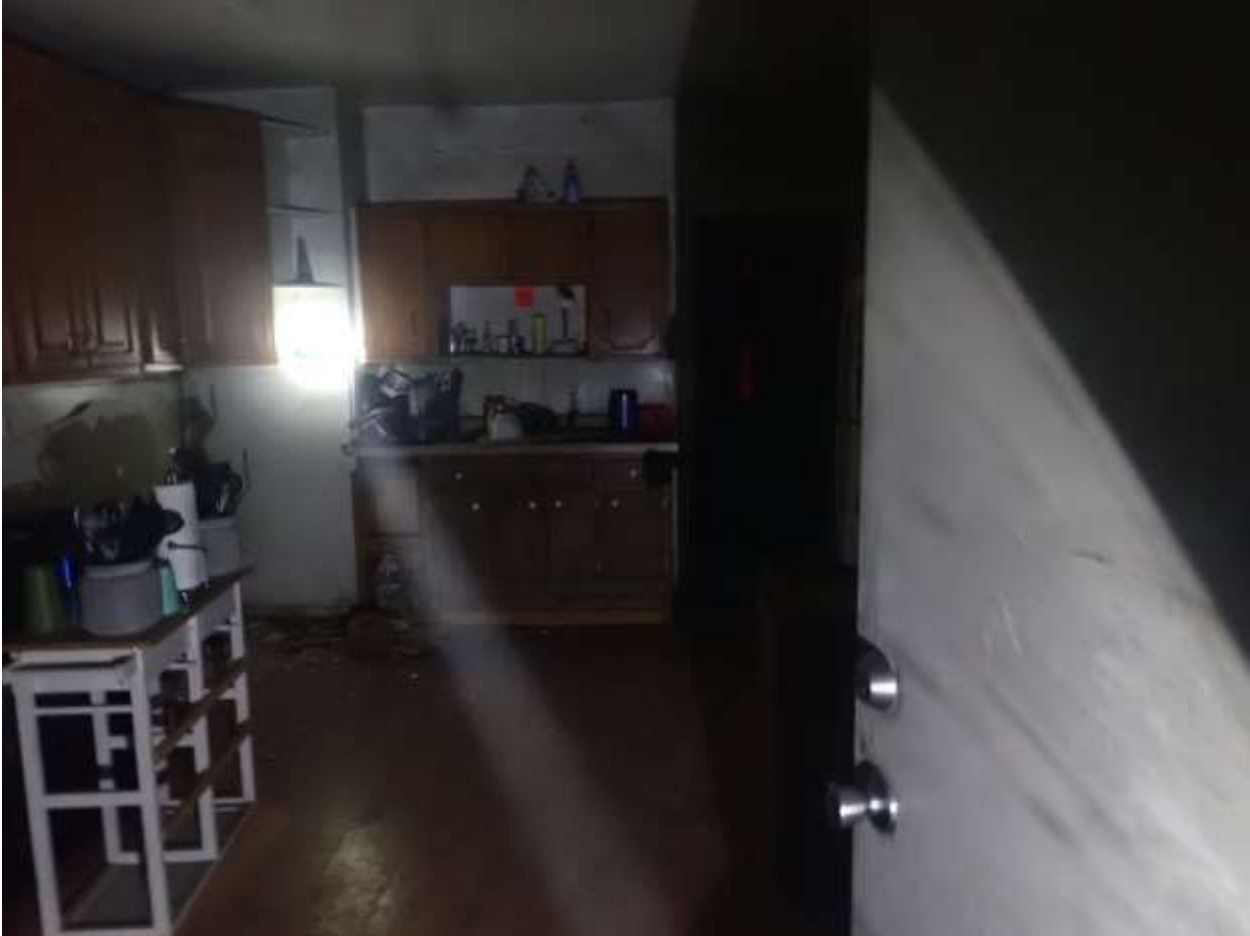
326 Charles Ave – Fire photos sent on 7/11/23
