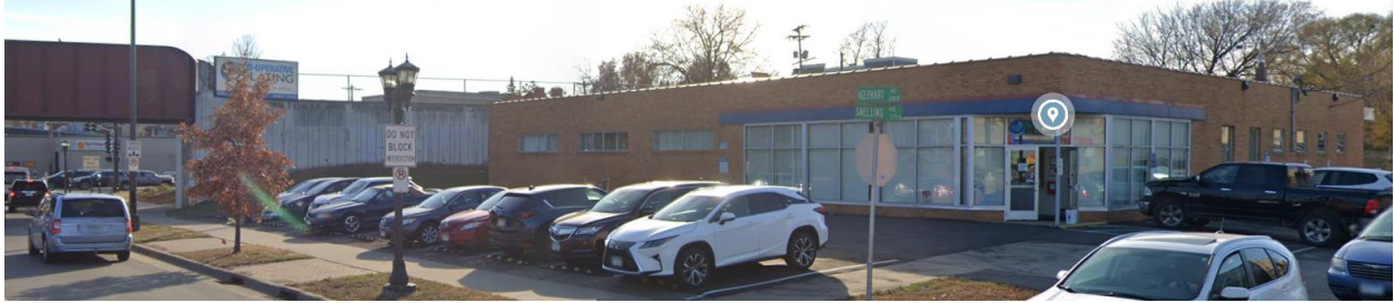
271 Snelling Avenue North, railroad and railroad bridge on the left
