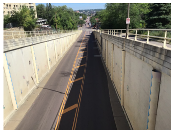
Robert Street Viaduct looking north.
