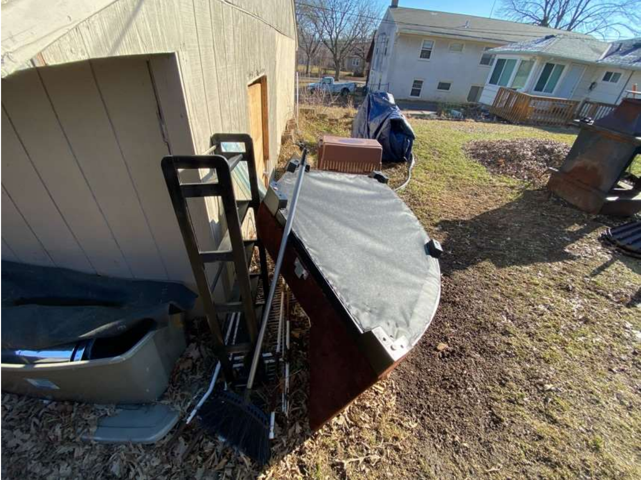
1823 7 th St E – rechecked photos 2-12-24
