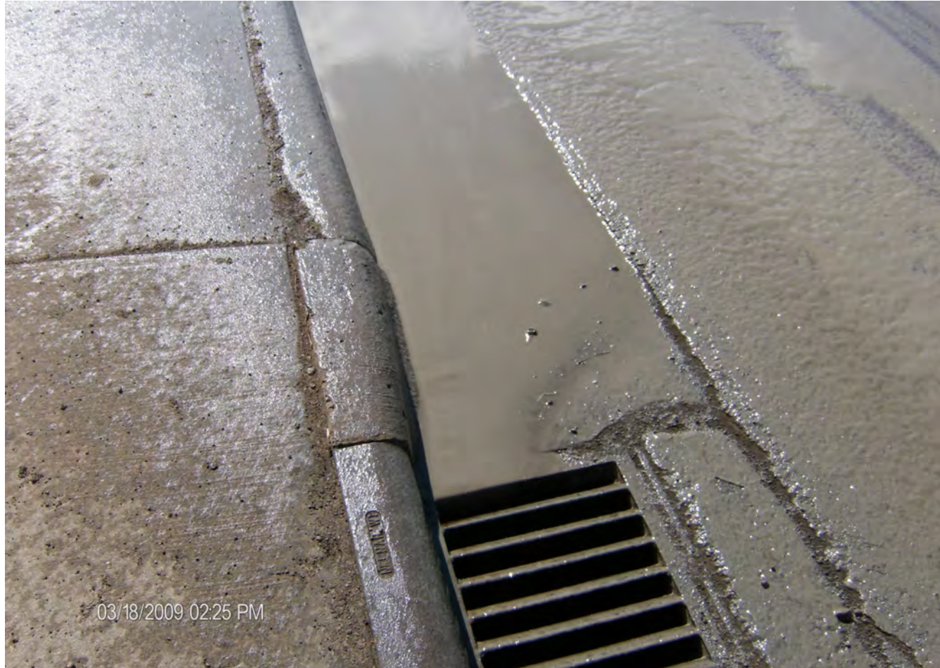
Discharge of Drilling Mud
