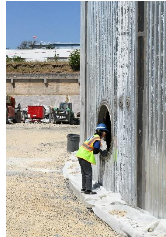
Che Fei Chen, Production Div. Mgr., looks through a manway in one of the clarifiers
