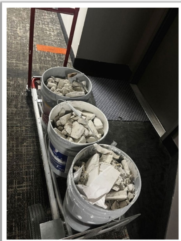
Carting uncovered suspect ACM drywall in hallways.
