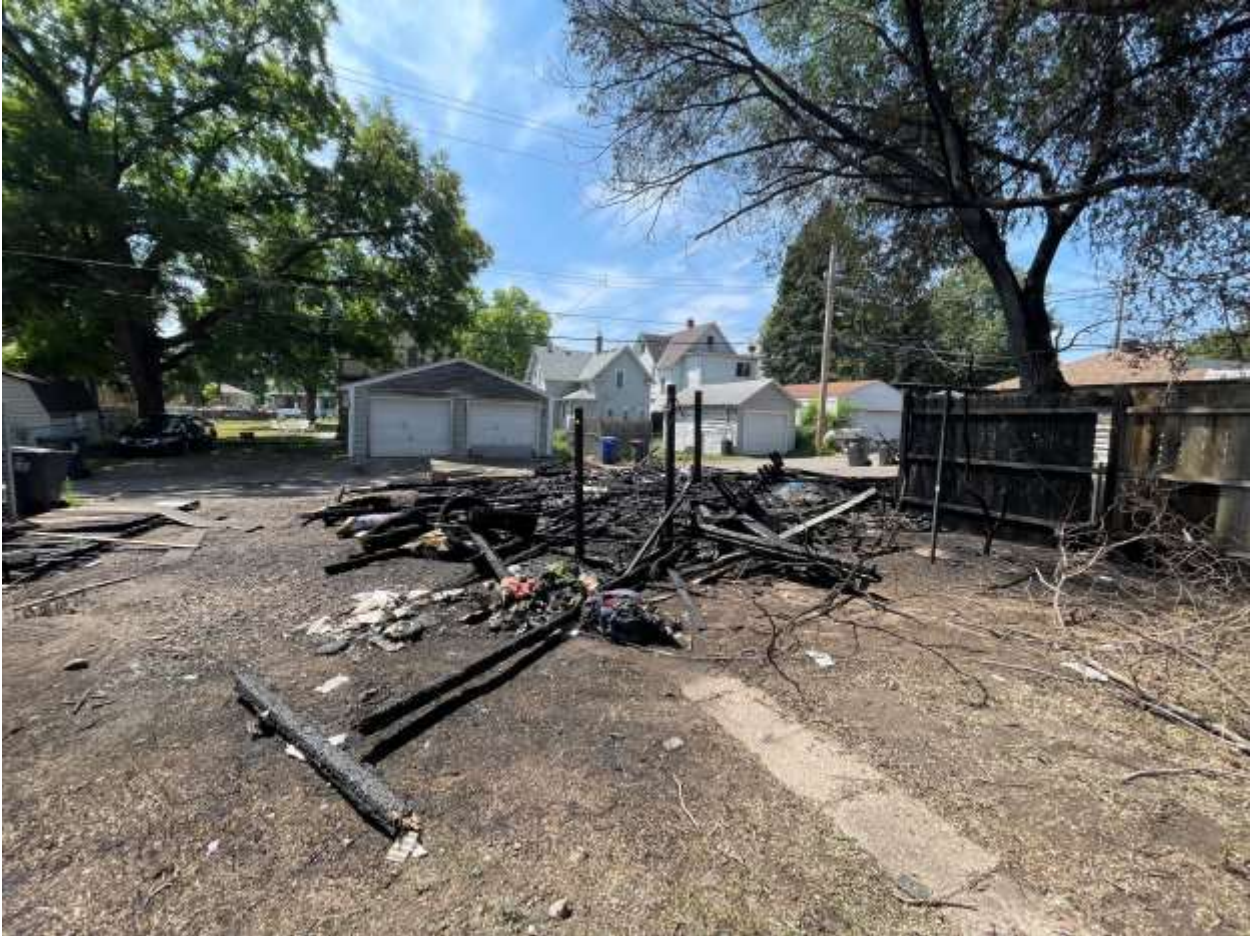
792 Rose Ave E. Garage fire 6/28/23
