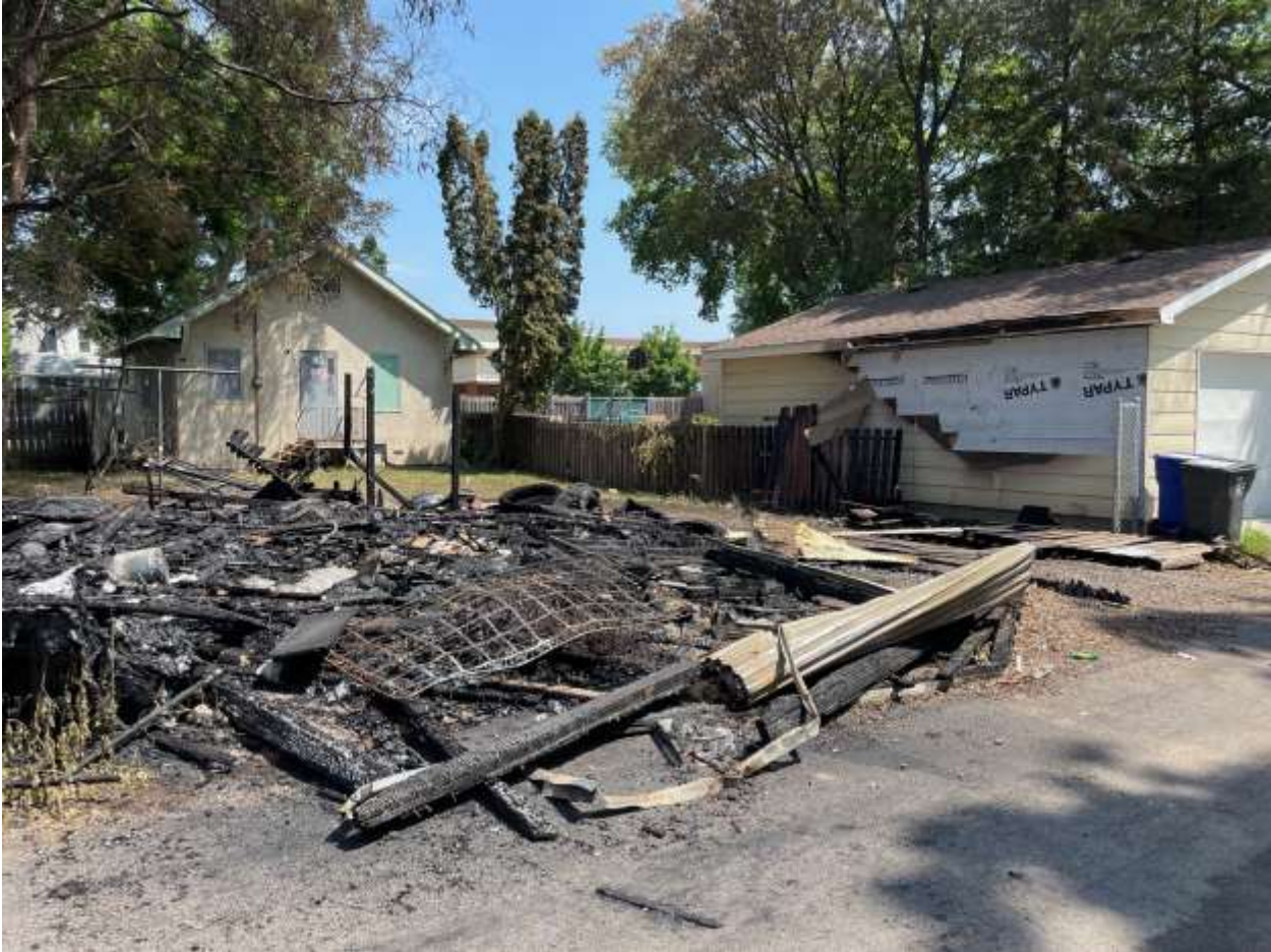
792 Rose Ave E. Garage fire 6/28/23
