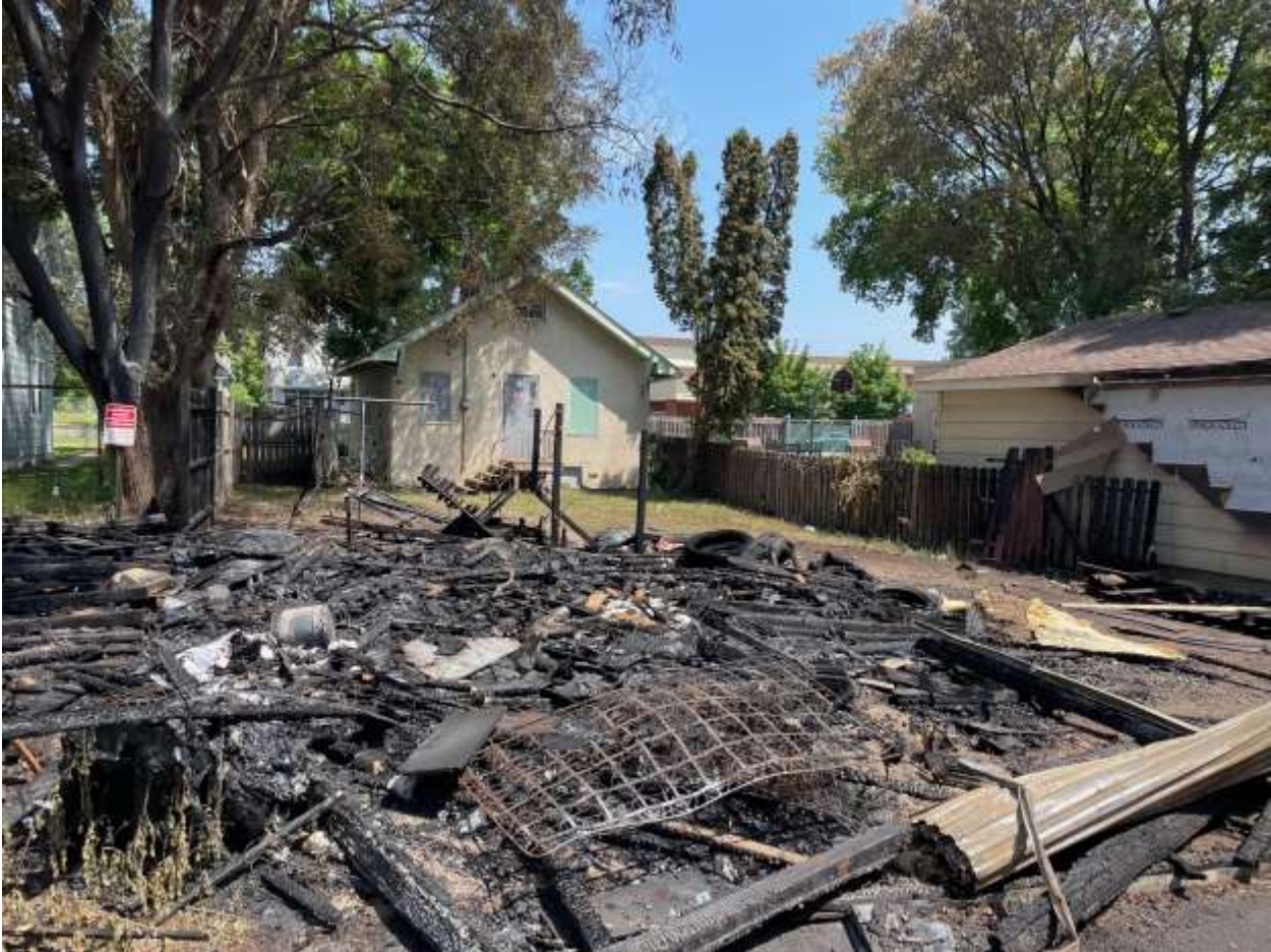
792 Rose Ave E. Garage fire 6/28/23
