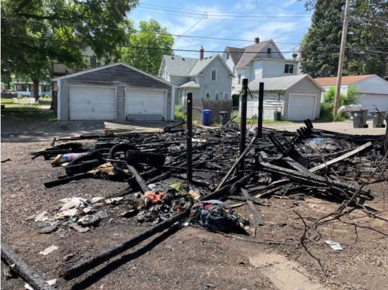
792 Rose Ave E. Garage fire 6/28/23
