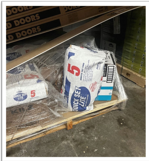
Renovation materials, including bifold doors and a joint setting compound, found in the Haven parking garage. Picture taken June 6, 2023.
