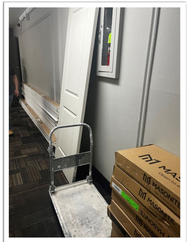
New baseboards and doors waiting for installation. Picture taken March 31, 2023.
