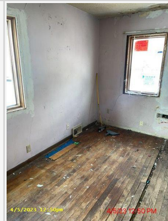
Photo: Before Photos - Miscellaneous - 0096_13_After_App- Relocate interior debris personals.jpg
