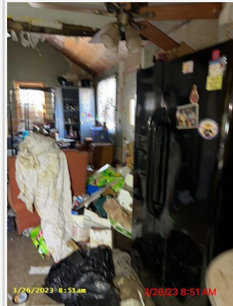
Photo: Bid Photos - Miscellaneous - 0008_Before_Condition - Interior.jpg Description: Bid Photos Description: ST0029866672
