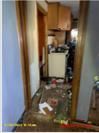
Photo: Bid Photos - Miscellaneous - 0003_Before_Condition - Interior.jpg Description: Bid Photos Description: ST0029866672
