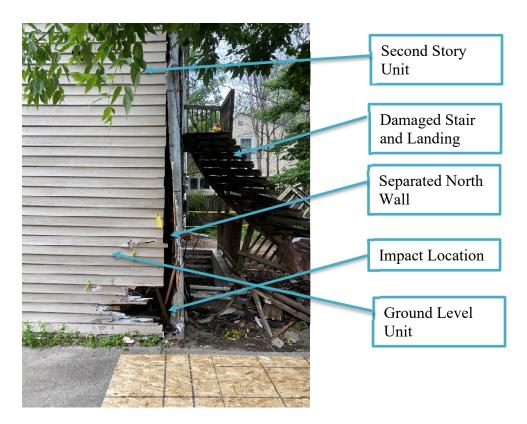
Damage to the structure appears to be as follows: Separated north building wall, dislodged and broken exterior stair and exterior landing.
