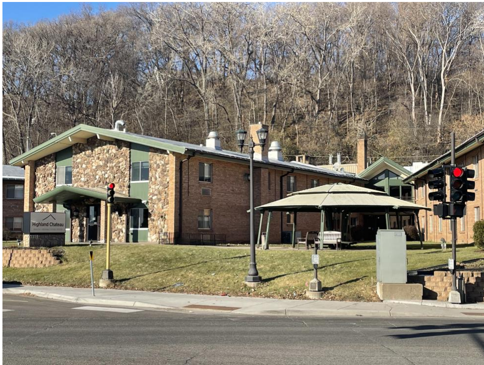
Photo 1- existing Highland Chateau (proposed development behind)
