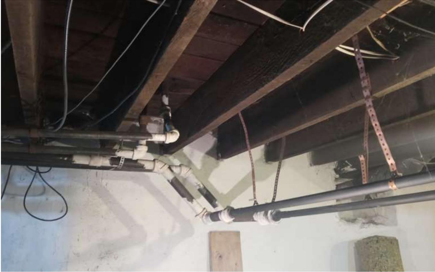
**Opposing Wall Pipes Strapped to Floor Joists**
