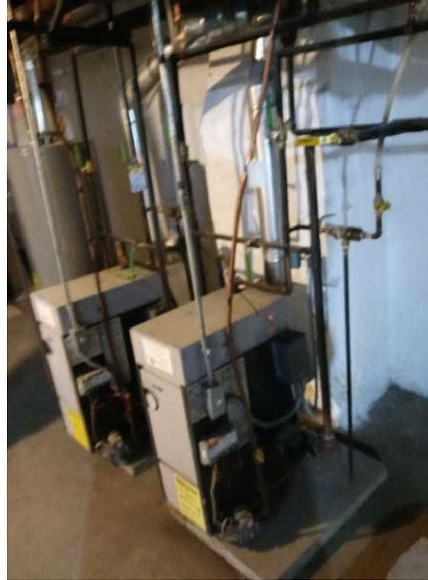
**Piping and Vents Strapped to Floor Joists**
