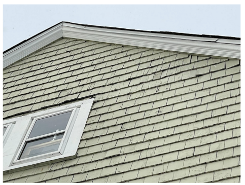
MATCH RAKE TRIM DETAIL FROM EXISTING HOUSE
