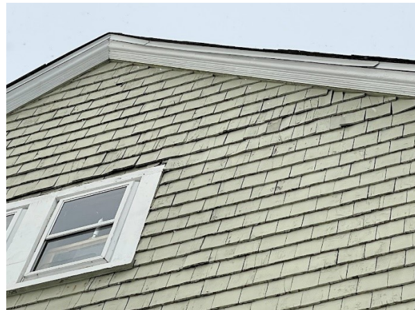
Figure 2 & 1. Existing predominate east facing gable end's shingle and rake trim details.
