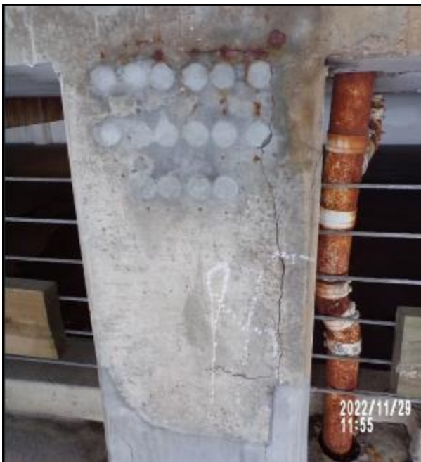
Level 2.5 previous column base patching starting to re crack
