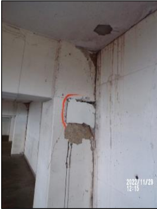
Column spall below beam at east foundation wall
