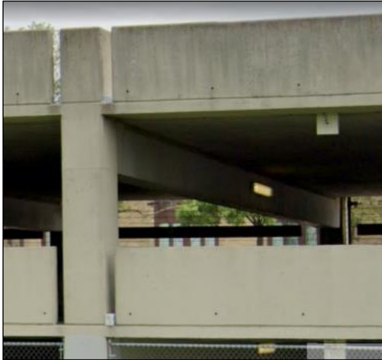
SK-2: Google Image of Level 3 ½ PT Beam
