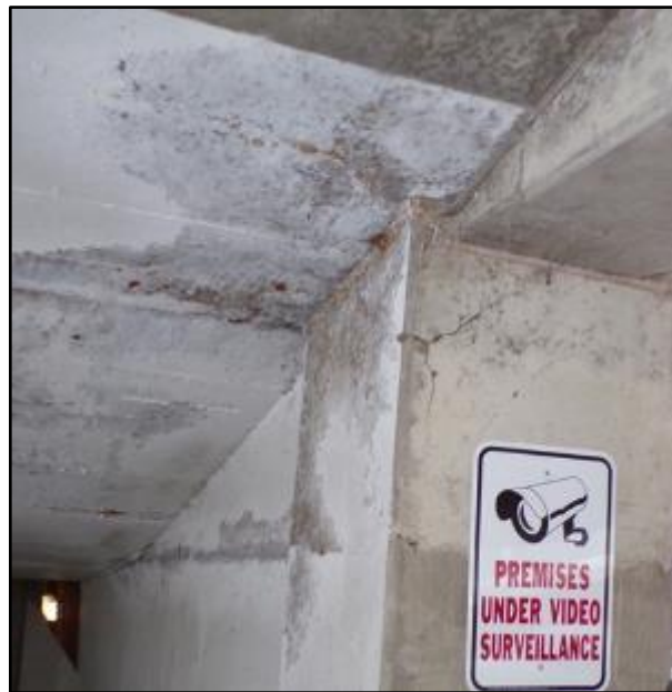
Column spall below beam at east foundation wall
