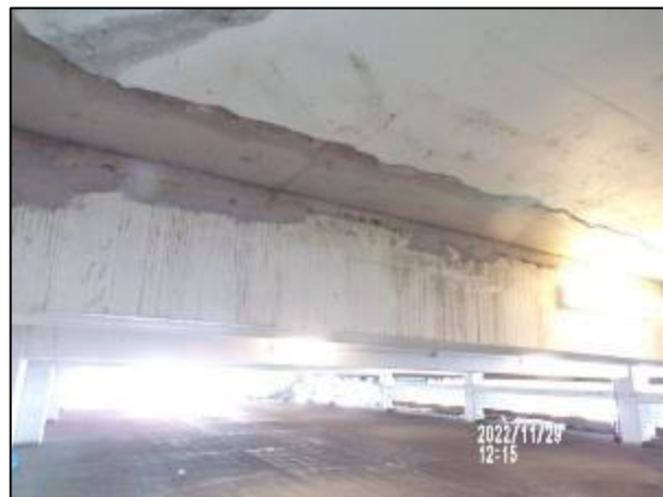
Previous patch full length of beams.
