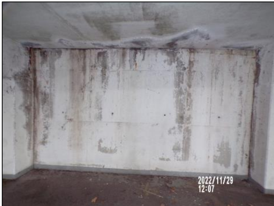
East foundation wall between beam supporting columns Grid C
