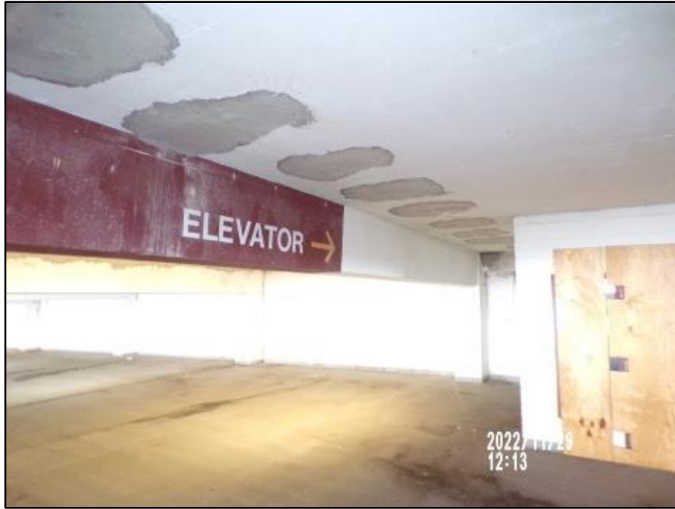
Previous bollard through bolt patching under Level 3.
