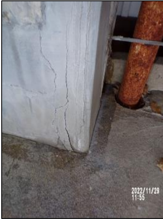
Level 2.5 previous column base patching starting to re crack
