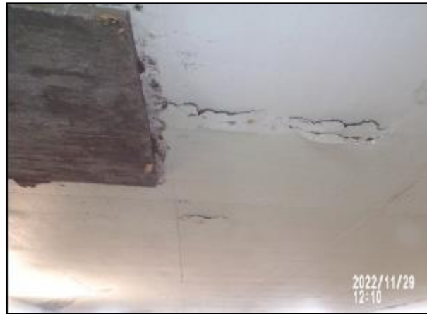
Left: Previous bottom of slab patch was formed lower than original bottom of slab. Right – Continued spalling next to patch.
