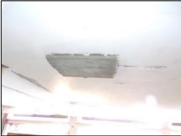
Left: Previous bottom of slab patch was formed lower than original bottom of slab. Right – Continued spalling next to patch.
