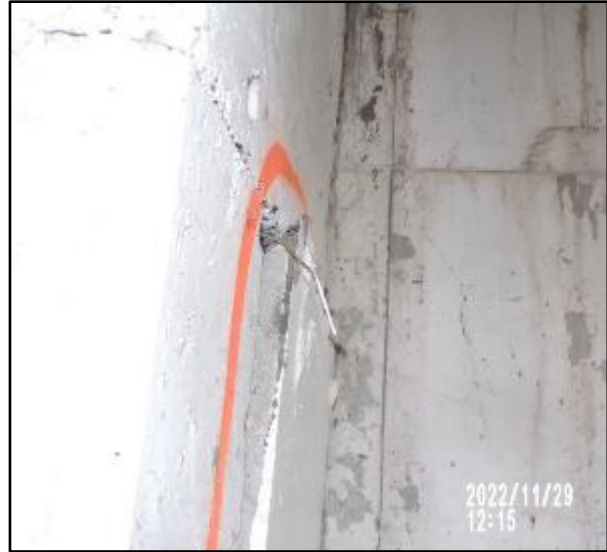
Column spall below beam at east foundation wall
