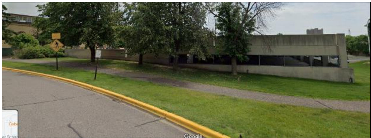
SK-8: Google Image of north end Levels 2½, and 3½. Note grade rising on east (left) end.
