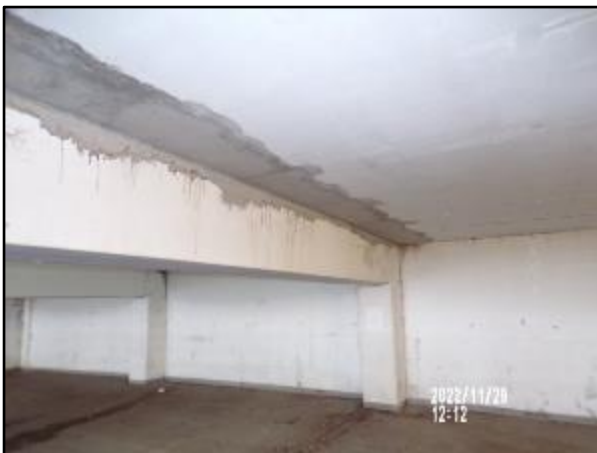
Previous patch full length of beams.
