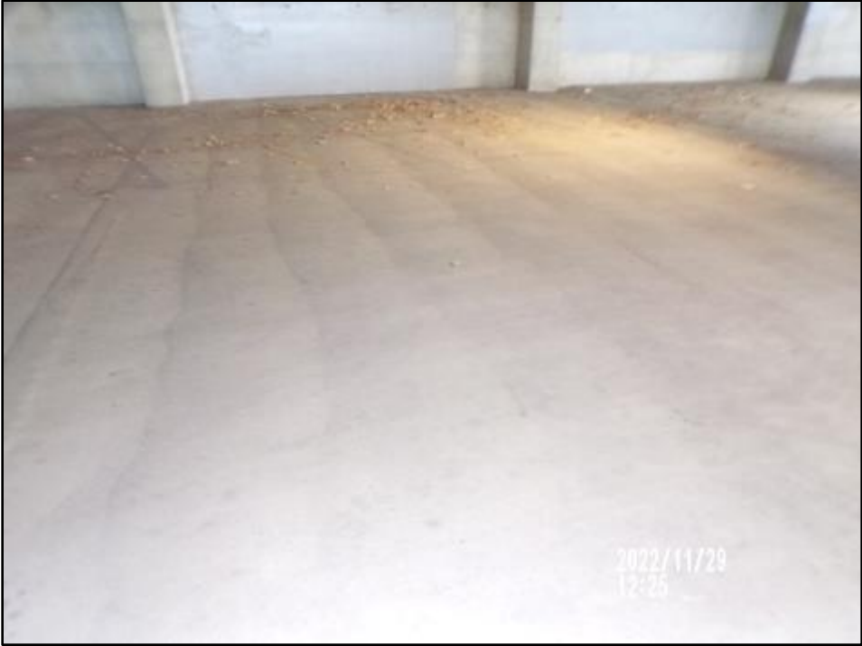
Level 1 slab on grade east side
