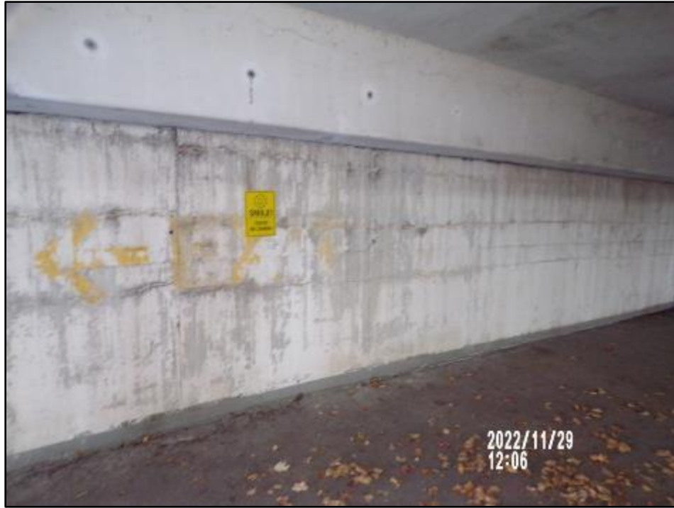
North foundation wall
