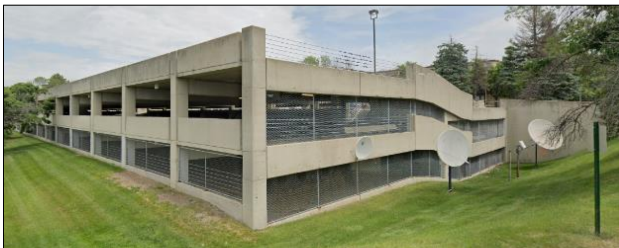
SK-6: Google Image of Southwest Corner of Levels 1 ½, 2 ½, and 3 ½ in foreground.
