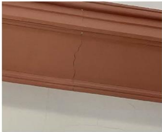
Plaster Cracking
