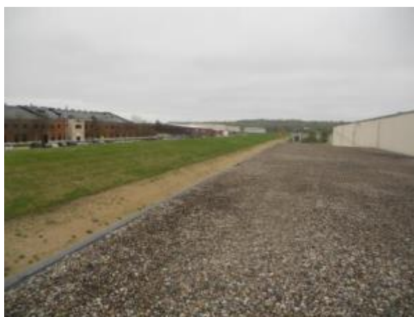
Levee West of 260 Building
