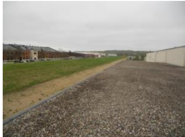
Levee West of 260 Building
