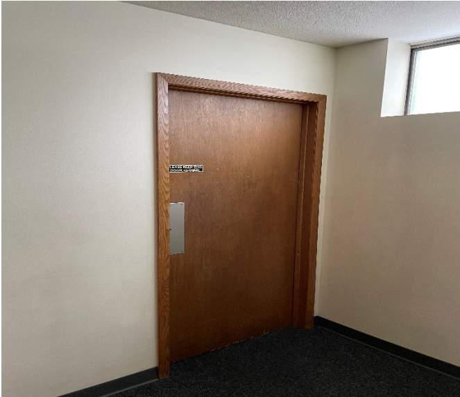
Door into 1 of 2 stairwells leading directly to exterior
