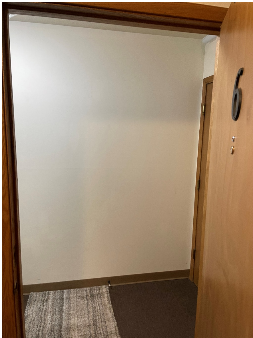
Hallway outside unit 6
