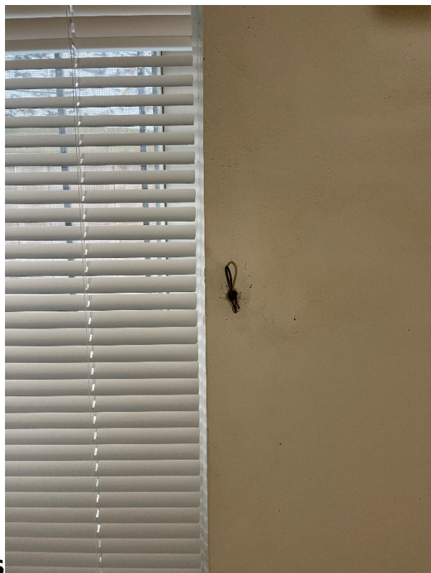
S Pin to release bars from window in unit 1.
