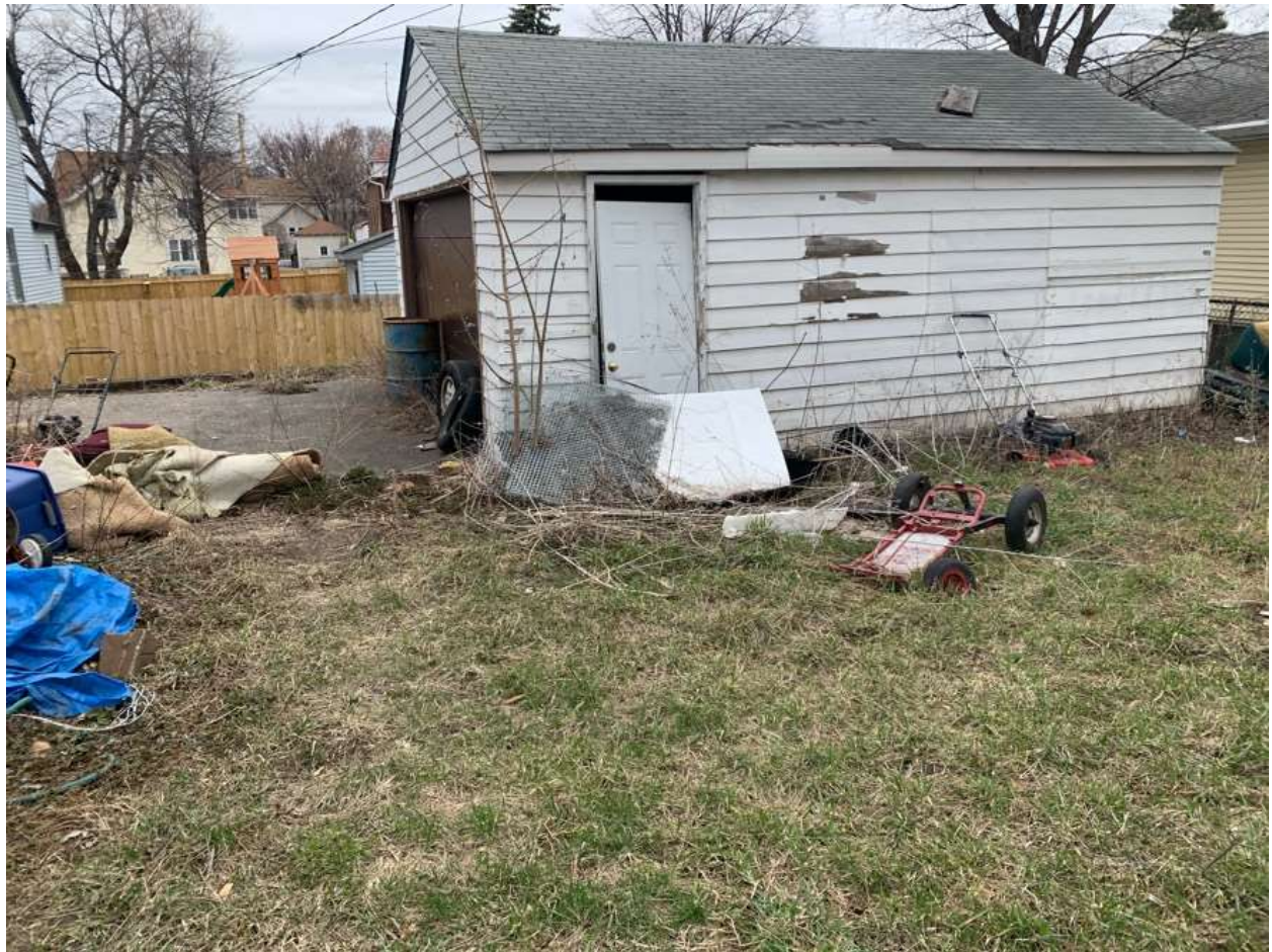
264 Earl St Photos taken on 4/28/22
