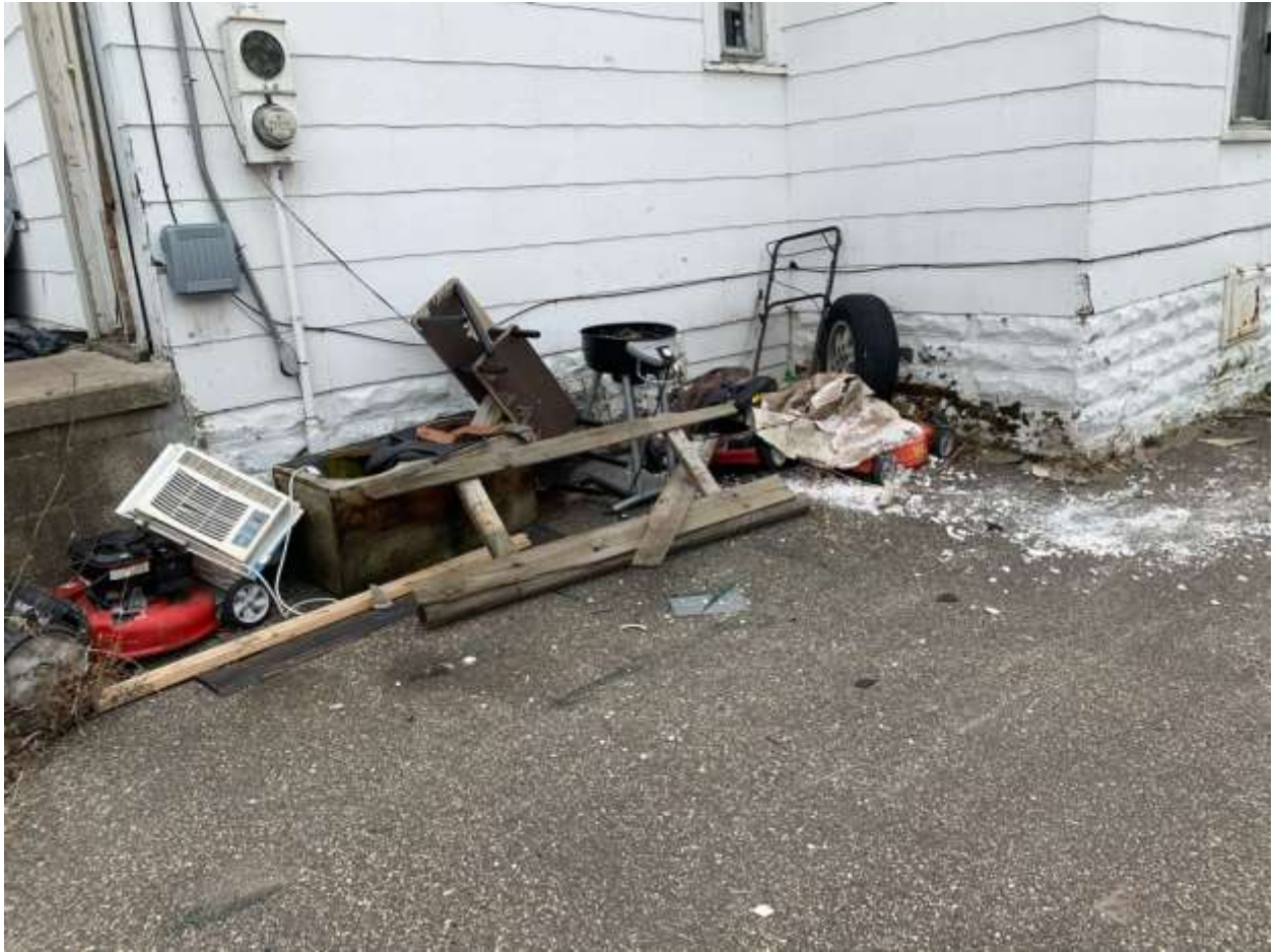
264 Earl St Photos taken on 4/28/22
