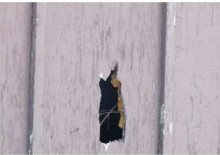
North wall deterioration and holes present
