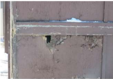
North wall deterioration and holes present
