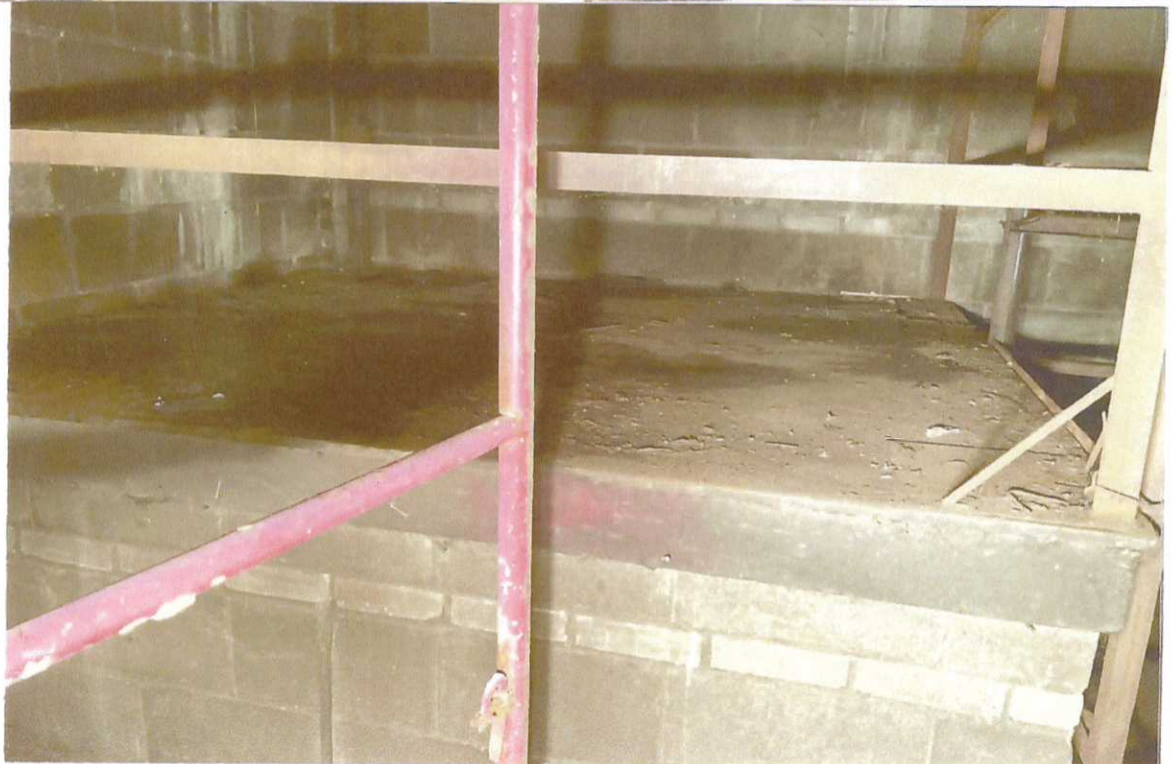
SW Mezzanine Cleared
