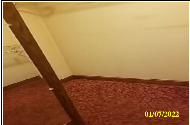
Date Serviced: 01/07/2022 Room: No Room Category: Interior Repairs
