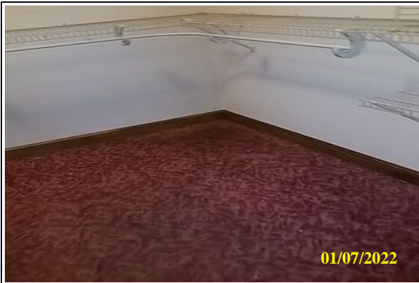
Date Serviced: 01/07/2022 Room: No Room Category: Other
