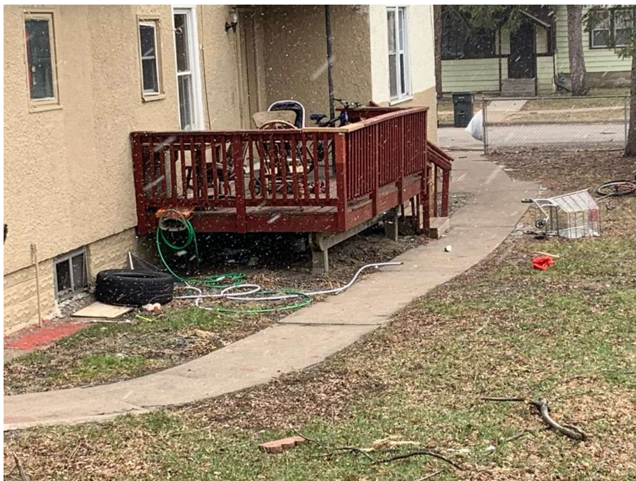
501 Hopkins St Photos rechecked on 4/15/22
