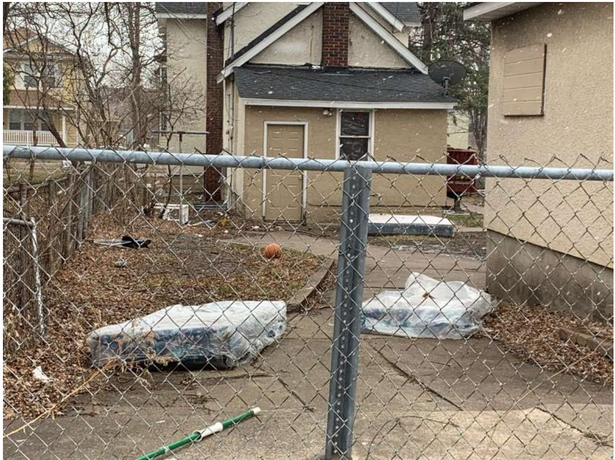
501 Hopkins St Photos rechecked on 4/15/22
