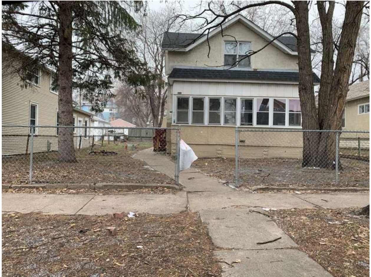
501 Hopkins St Photos rechecked on 4/15/22
