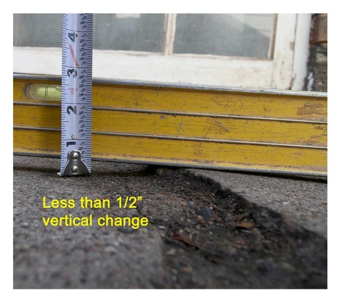
This measurement is irrelevant as private sidewalks are not regulated by building code. Nonetheless it shows that with very minor repair this sidewalk would comply with industrial/commercial handicapped accessibility standards.
