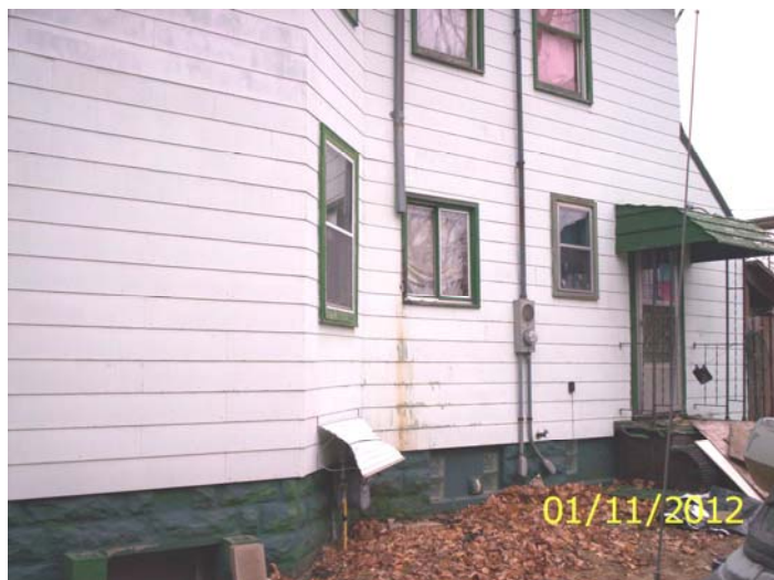
Rain leader drains over wall and at foundation
