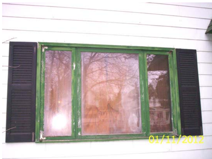
Rot damaged window, water staining on interior side of window
