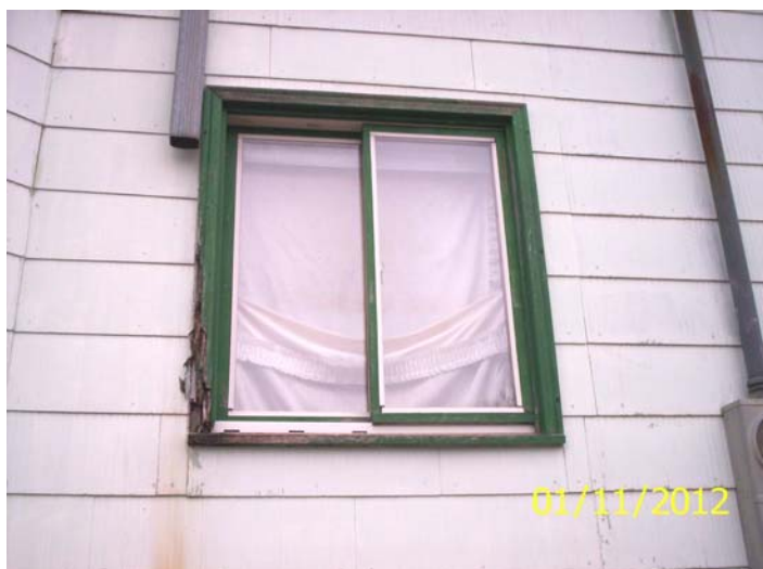
Rot damaged window, rain leader drains onto window
