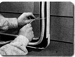
Attach the SpeediChannel™ to the base.
