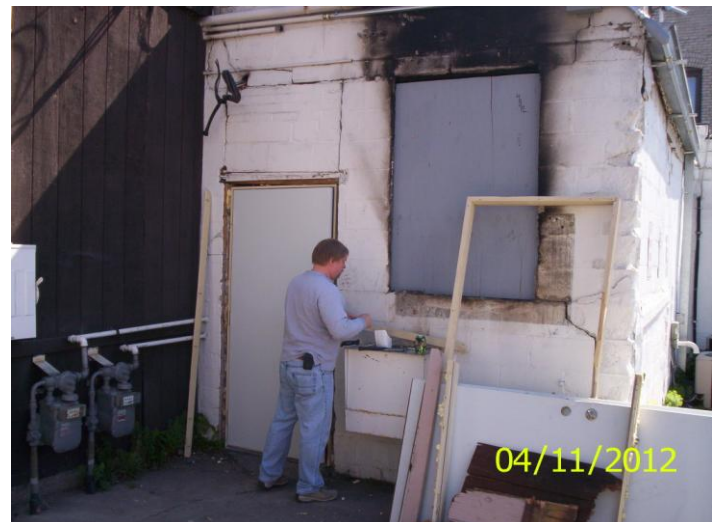
South side door and window
