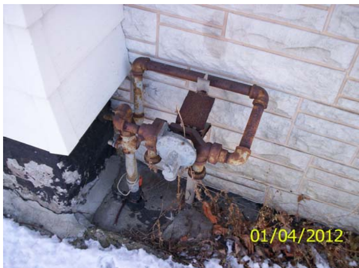
Gas meter removed
