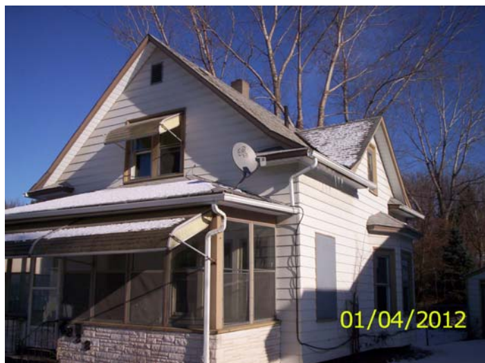
West and south side
