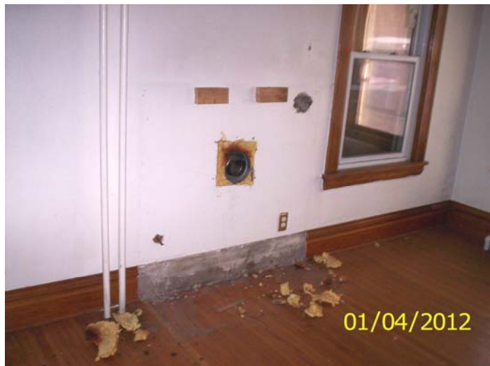
Missing floor board, missing wall mounted heater, open Wall, cut gas line for heater
