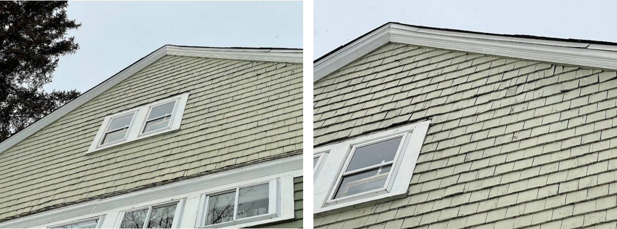
Figure 2 & 1. Existing predominate east facing gable end's shingle and rake trim details.
