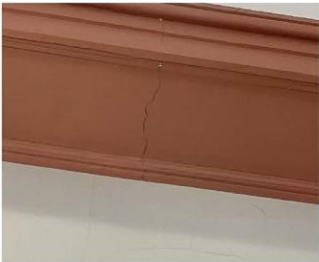
Plaster Cracking
