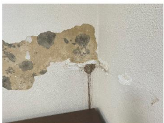
Water Damage in community room
