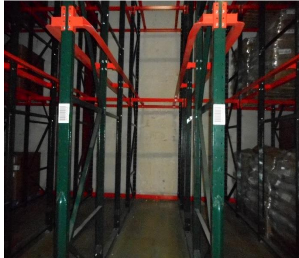
260 Building Freezer Wall – Exposed Expanded Polystyrene
