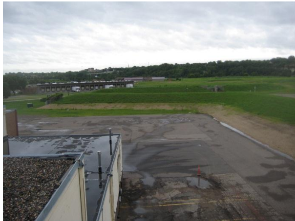
Levee Looking North from 240 Building
