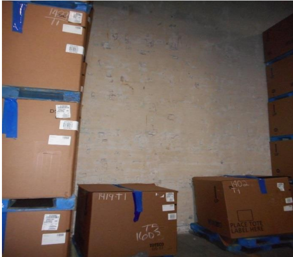
240 Building Freezer Wall – Exposed Expanded Polystyrene
