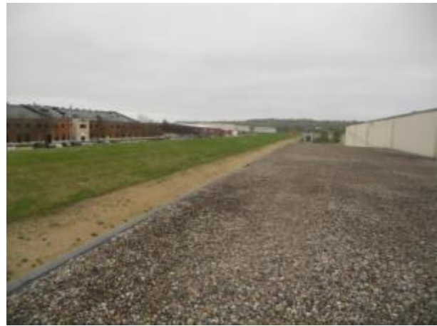
Levee West of 260 Building
