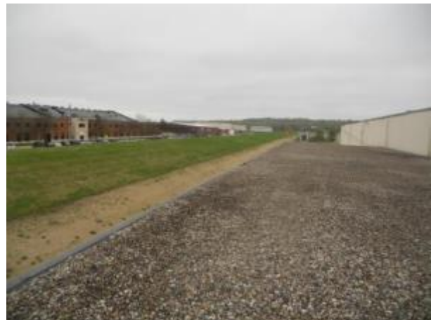
Levee West of 260 Building
