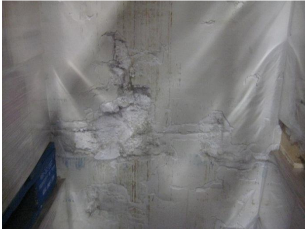
Freezer Wall – Exposed Expanded Polystyrene
