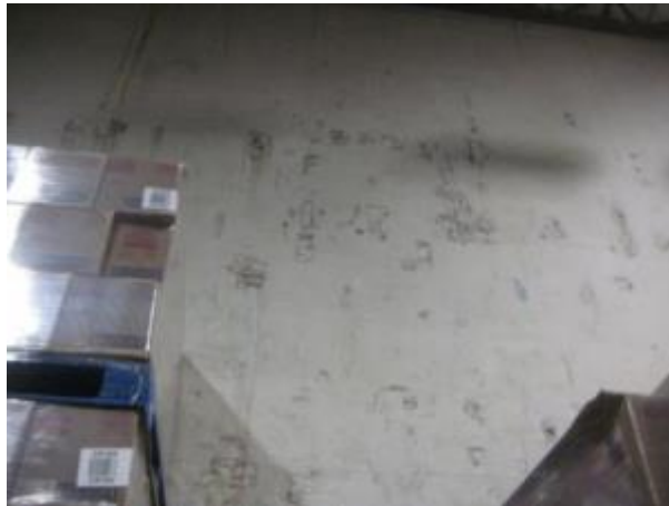
Freezer Wall – Exposed Expanded Polystyrene
