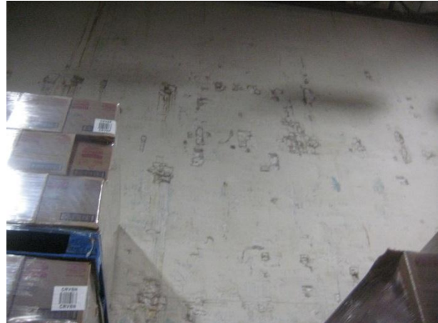
Freezer Wall – Exposed Expanded Polystyrene
