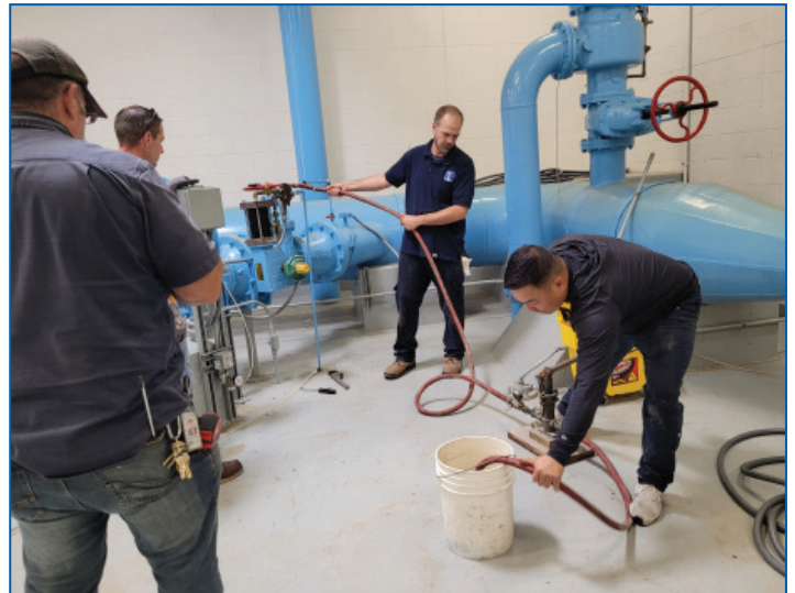
James Lee, maintenance worker, hand pumps to open the discharge valve at the Beebe Road pump station while Jon Hendrickson, Dick Keeney and Jon Falardeaux provide support.
