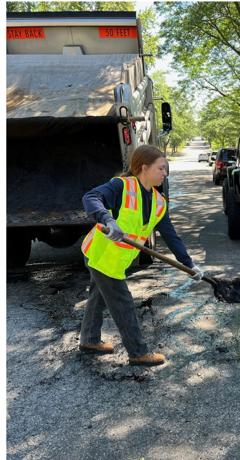
Pothole Filling with Public Works
