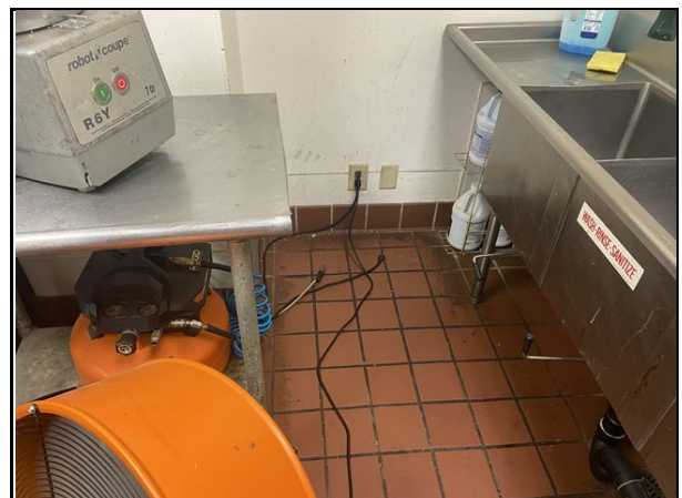
18 No structural issues noted in visible portions of eastern wall of building.
