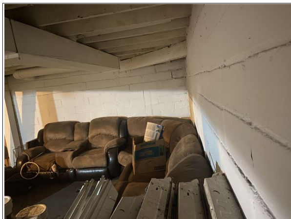
15 No structurally significant displacement noted in eastern foundation wall in basement.
