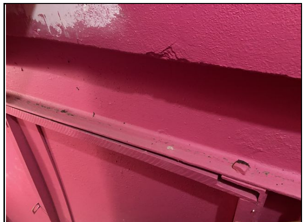
24 Existing framing in basement in good condition.
