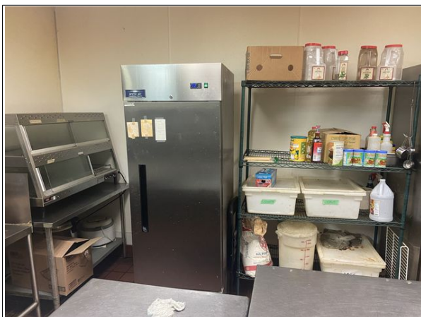
17 No structural issues noted in visible portions of eastern wall of building.
