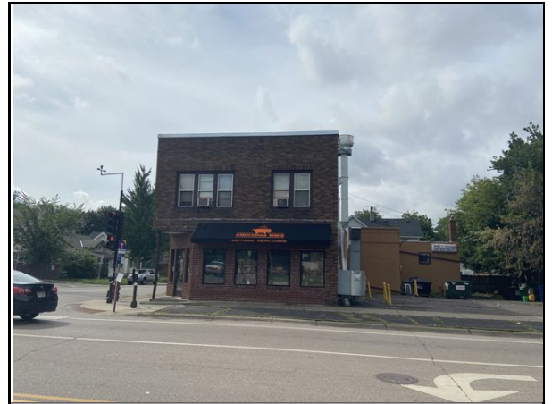
2 North side of building.
