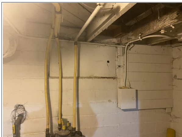
9 No structural issues noted at eastern foundation walls in basement.
