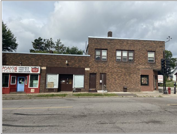
1 East side of building.
