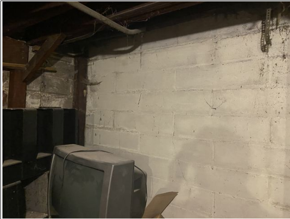
19 No structural issues noted in eastern foundation wall
