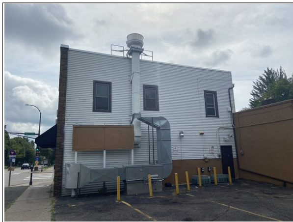
3 West side of building.
