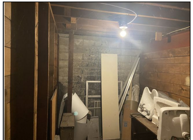
22 No structural issues noted in eastern foundation wall.
