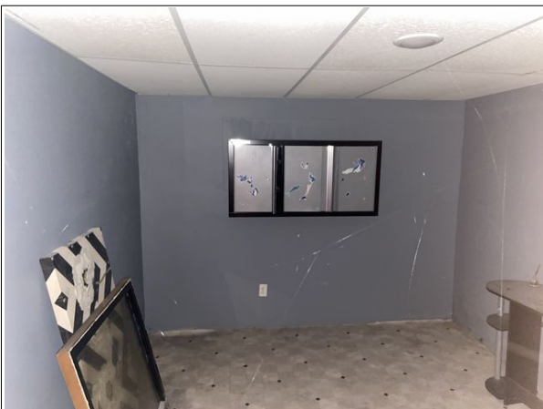
23 No structural issues noted in finished portions of basement.
