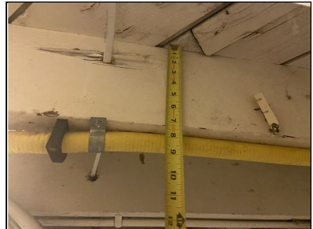
14 First floor joists in overall good condition.
