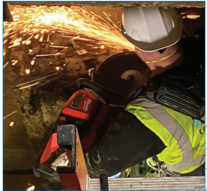
Photo by Steve Neil, Jacobs Engineering
