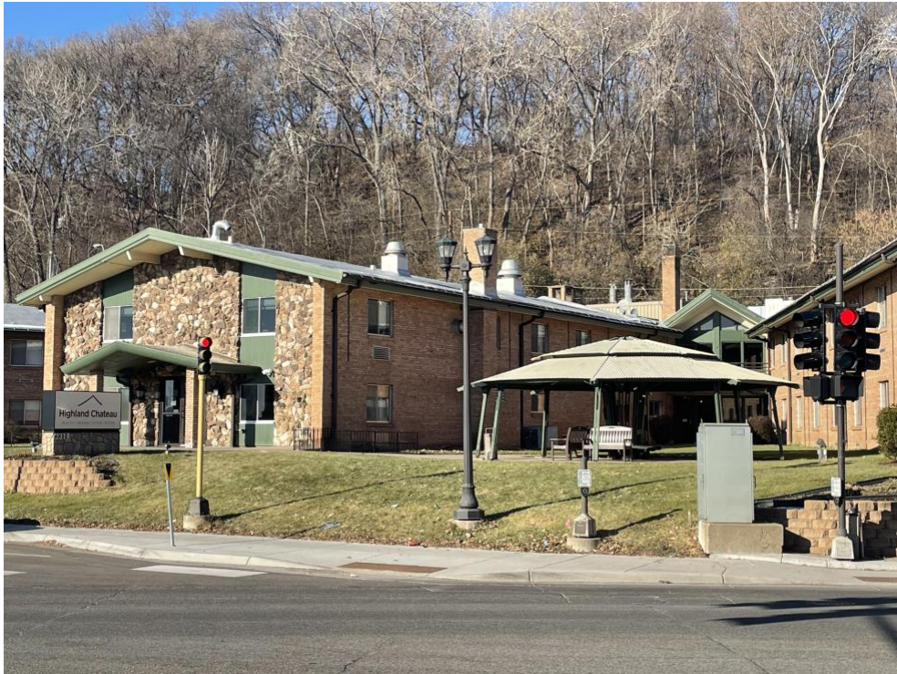
Photo 1- existing Highland Chateau (proposed development behind)
