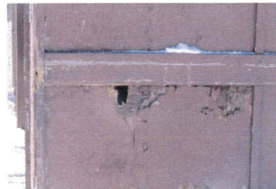
North wall deterioration and holes present
