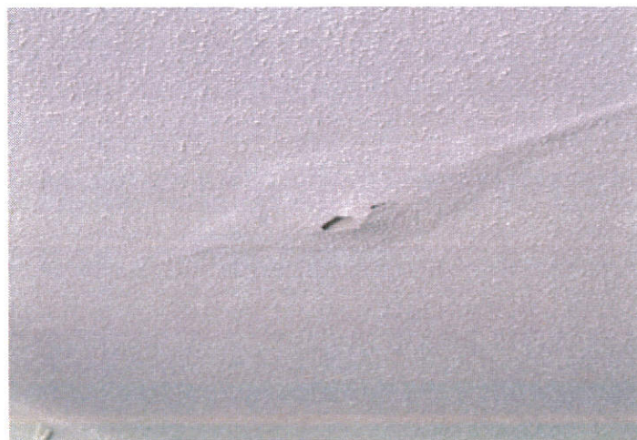
North wall deterioration and holes present
