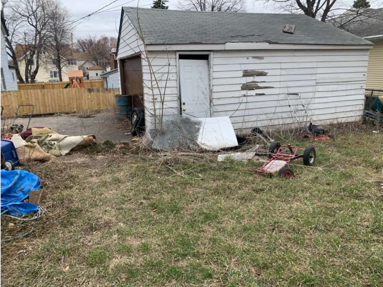
264 Earl St Photos taken on 4/28/22
