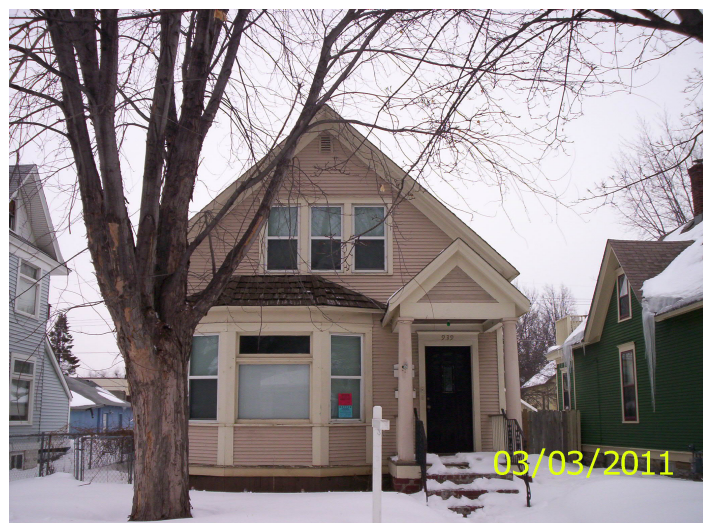
South side, posting
