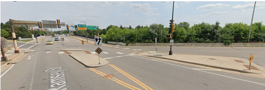
Right of way to the south – Pleasant, Grand, Ramsey, Grand Hill, Interstate 35E below
